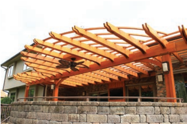
Cantilever structure with curved purlins which mirror the patio railing below
