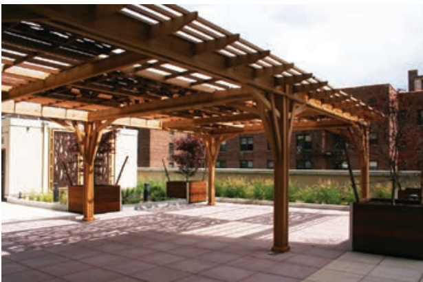
Large 18' x 36' pergola which frames several parasoleil panels providing shade and interesting patterns on the patio
