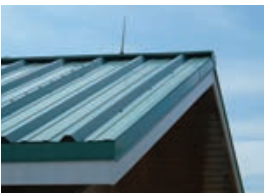
Lighting Protection Lightning rods, cable and grounding equipment
