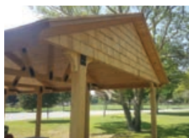
Cedar Glulam Frame Alaskan Yellow Cedar can be used on most shelter frames
