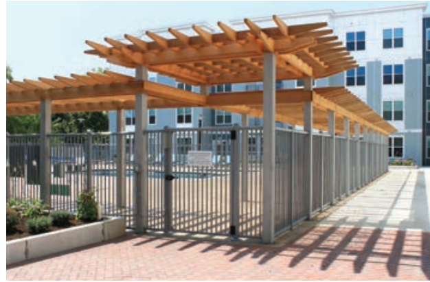
A dramatic pergola employing aluminum posts and beams supporting a dense rafter layout in quadrants
