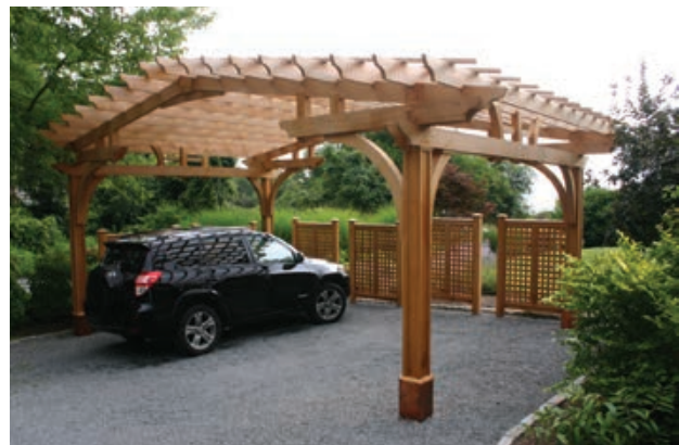
Carport pergola created to span up to 22'; also employs privacy lattice panels that are freestanding and used as a visual divider
