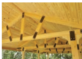
Cedar Roof Decking #1 grade, kiln dried 2" x 6" Alaskan Yellow Cedar
