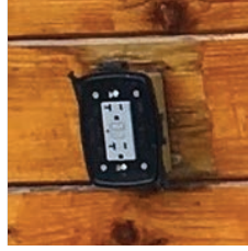
Outlets or GFCI Outlets Per plan
